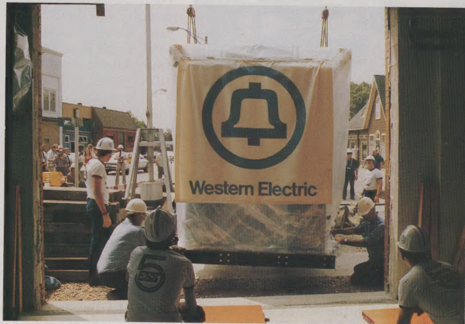
Left — The 22 ft. by 6 ft. by 8½ ft. switch is lowered to ground level at the Illinois Bell office while the whole town watches. Below — The 13,600-pound "package" inches by the town's flagpole.
